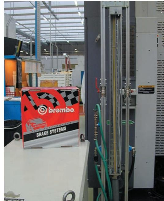
Another advantage of the Teseo system is the complete absence of rusting and contamination inside the HBS profiles, reducing the cost of air treatment and prolonging the life of tools and downstream equipment. Also the absence of air leaks due to the positive 'O' ring seals reduces energy costs for the airmain system.
